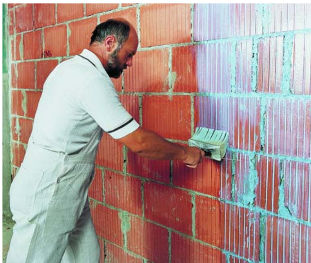
PCI Gisogrund helps improve adhesion of plaster and lime plastering to brickwork.
