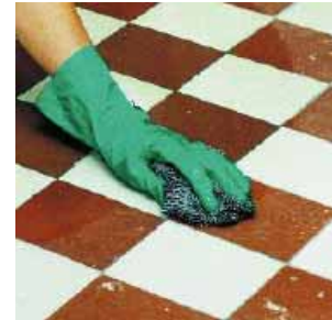
Remove bond-breaking residues from the substrate using a suitable cleaning agent (e.g. PCI Univerdünnner).
