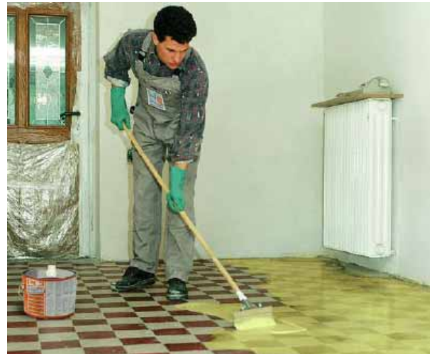
PCI Gisogrund 303 is the secure primer for laying coverings on ceramic tiles.
