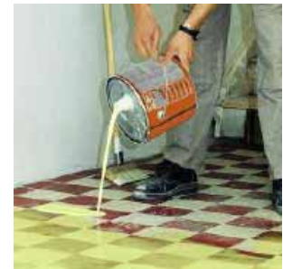
Shake PCI Gisogrund 303 well before use and pour onto the substrate.
