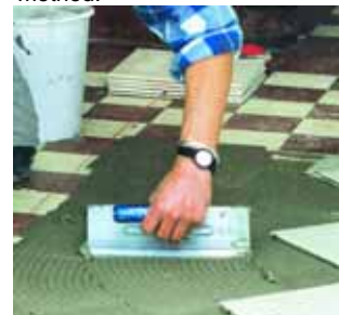
Subsequent top coverings can be installed after approx. 3 hours.
