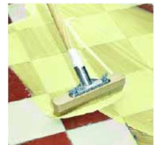
Spread primer over the substrate working in criss-cross method.
