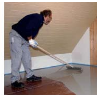
and de-aerated with a spiked roller.
