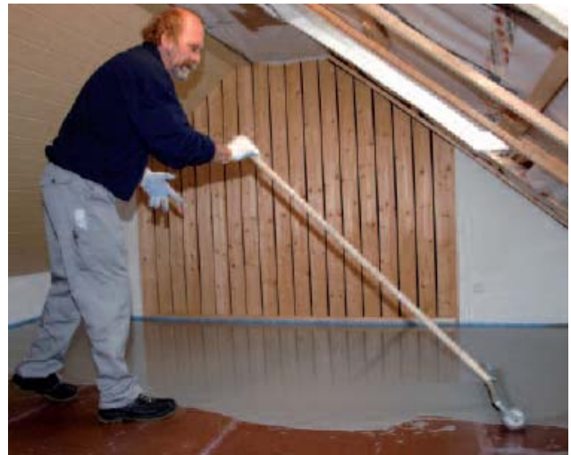
PCI Nanosilent helps reduce the impact sound and isolate the substrate in one application.
