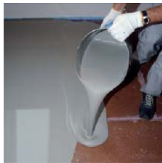
PCI Nanosilent is poured on to the substrate...
