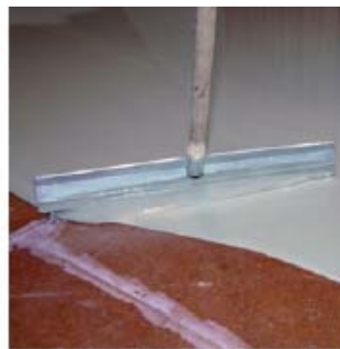
spread to the required thickness with a suitable surface scraper...
