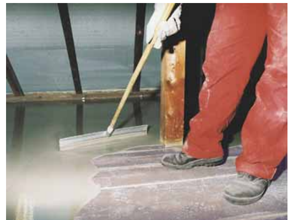
Fibre-reinforced PCI Periplan extra is especially suitable to level timber and chipboard floors in renovation and refurbishment works.
