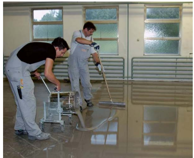
The very good self-levelling properties of PCI Periplan fein enable the application by surface scraper in upright position for efficient and very smooth levelling of floors.
